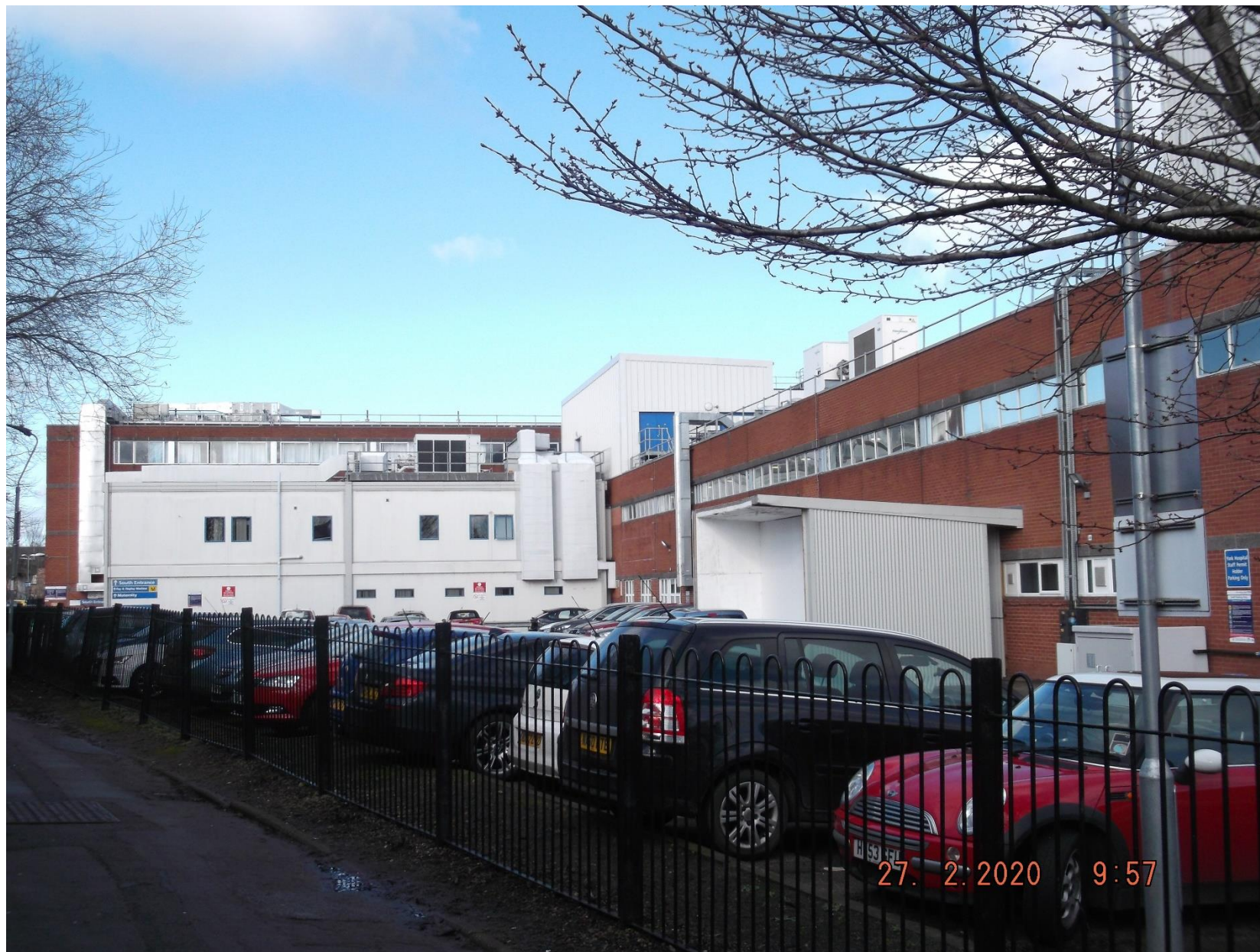
Site from Bridge Lane (2)
